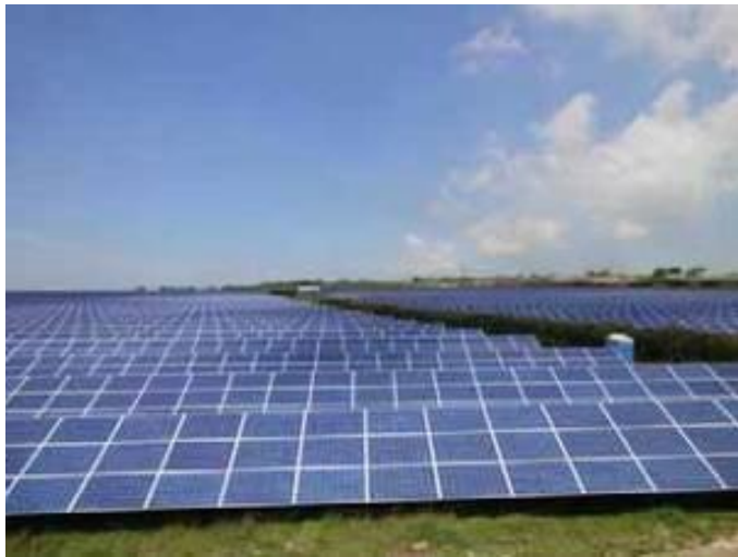
The 5MW Trefullock solar PV farm, Cornwall
